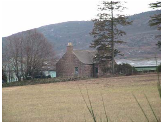
Fig. 4 : Existing farmhouse at Galton
