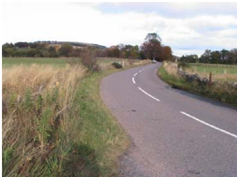
Fig. 5 : visibility to NE of access lane
